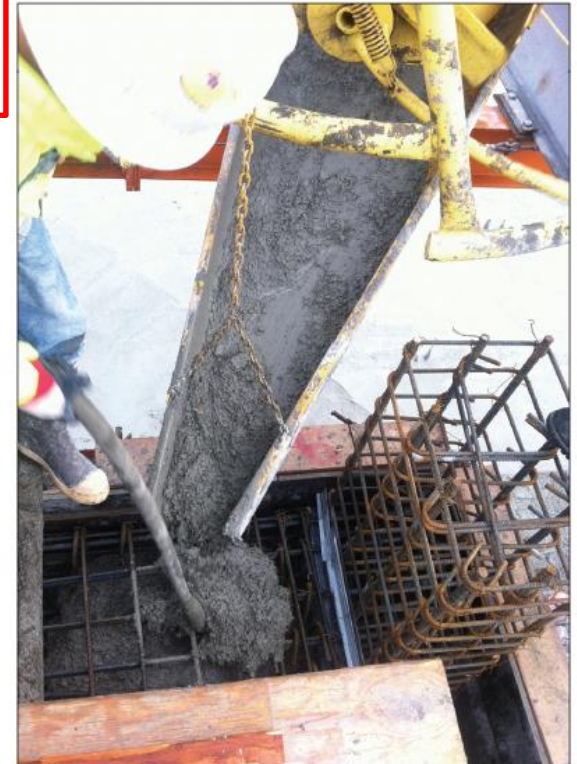
The city required two peer reviews before it would accept the new technology. Photos courtesy of Cary Kopczynski & Co.
