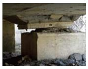
Figure 4: Displacement and damage to supports
