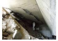
Figure 3: Damage to the outer box girder
