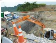
Figure 5: Repair of the abutment back wall
