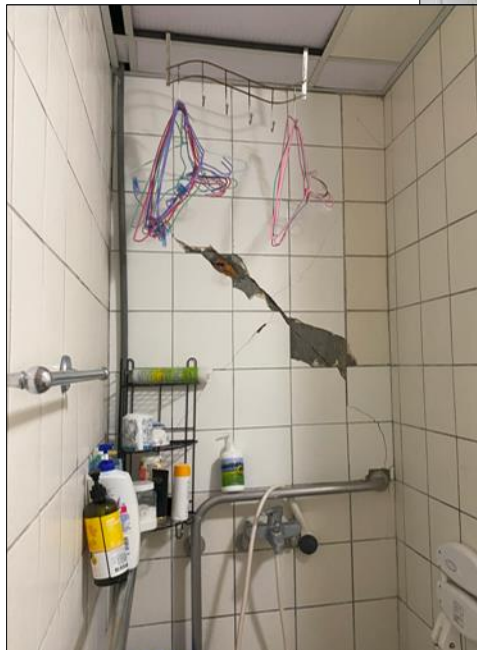
Cracked tiles on the opposite side of the wall
