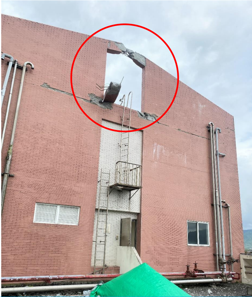
A beam connected to decorative gables collapsed on the penthouse
