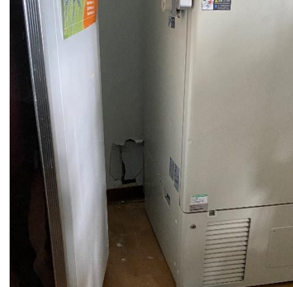
Partition wall damaged due to the displaced refrigerator
