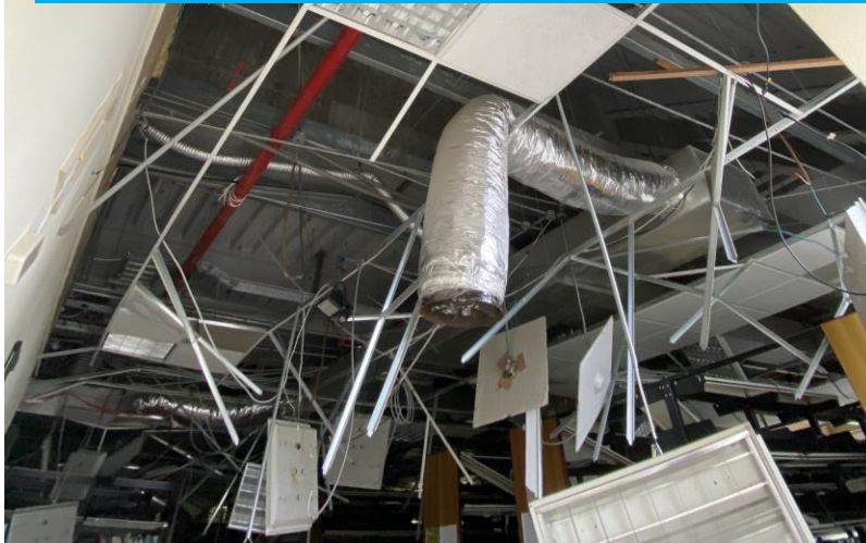
Damaged ductworks (6F of Bldg. DL)
