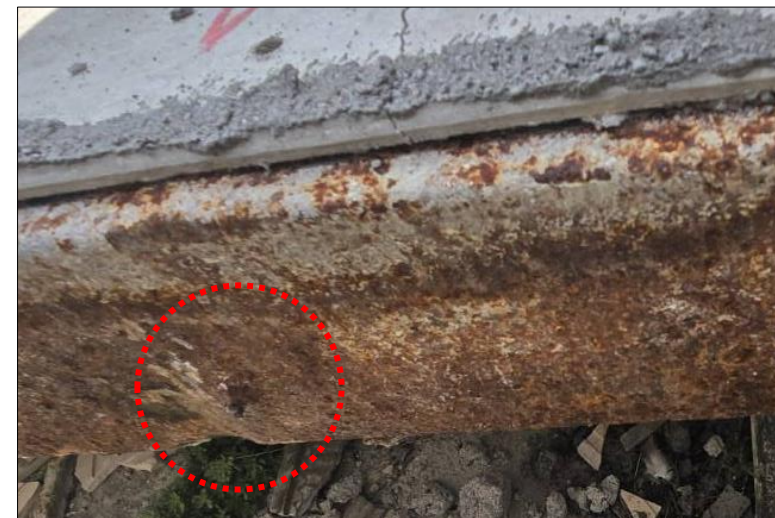
Failed anchorage of the collapsed wall
