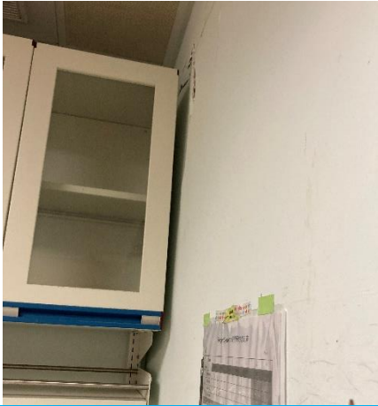
Partition wall damaged due to the tilted furniture
