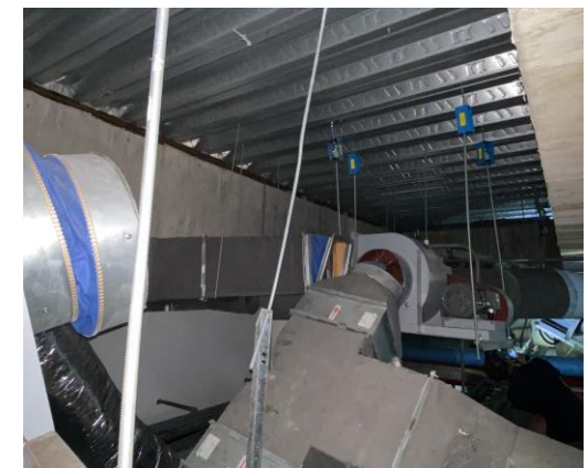
Separated ventilating machine and ductworks
