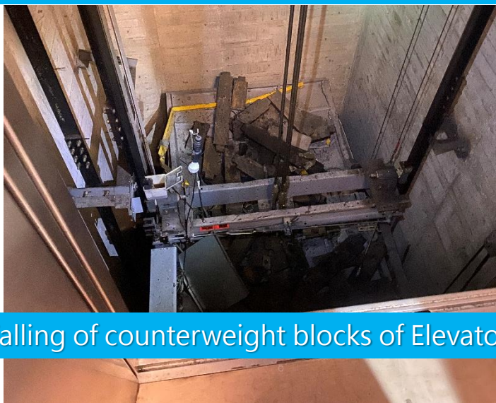
Falling of counterweight blocks of Elevator C
