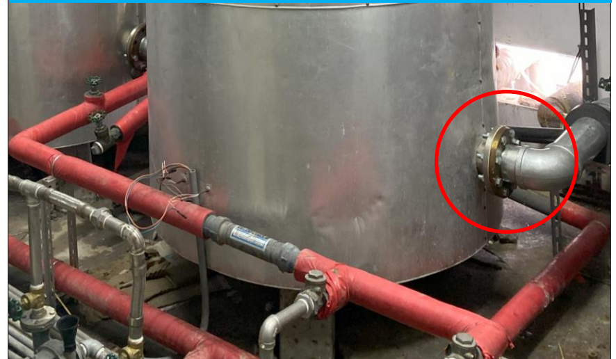
Damaged piping joints connected to the hot water tank in Bldg. A3 (repaired)
