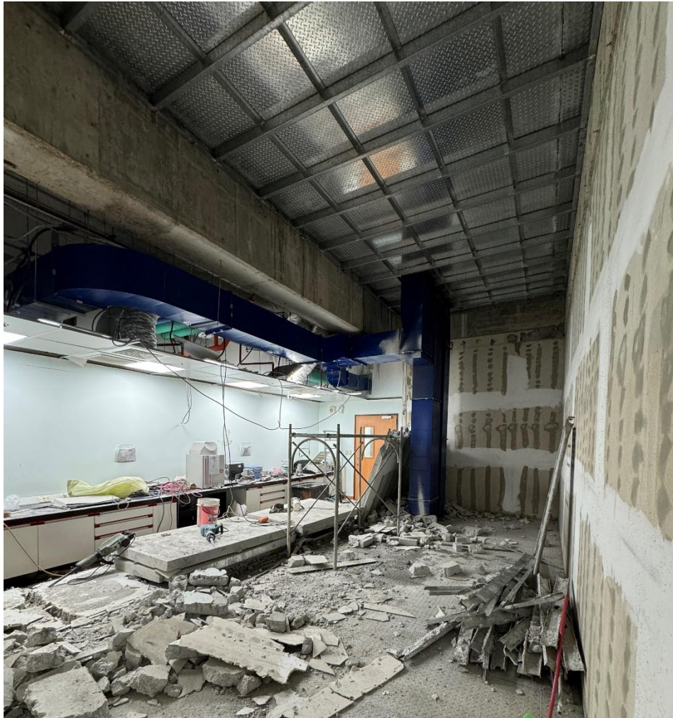
Tilted lightweight aggregate concrete (LWAC) walls (6F & 8F)
