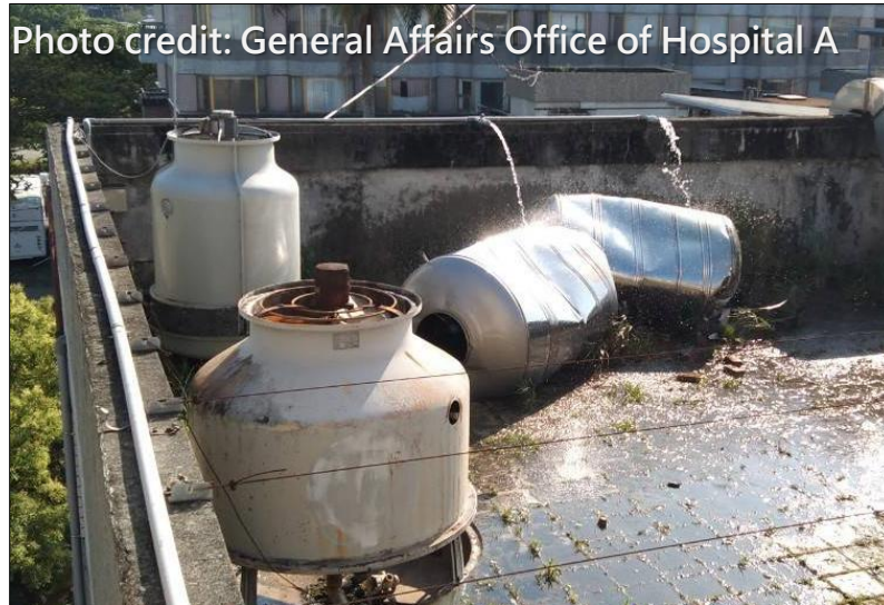
Collapsed tanks at rooftop of Bldg. A1
