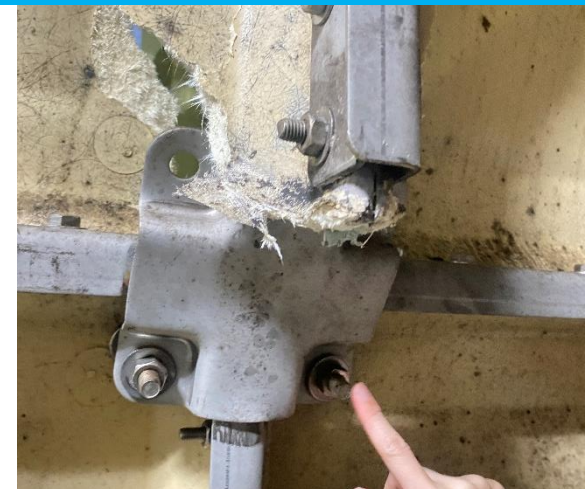
Damage to the connection joints
