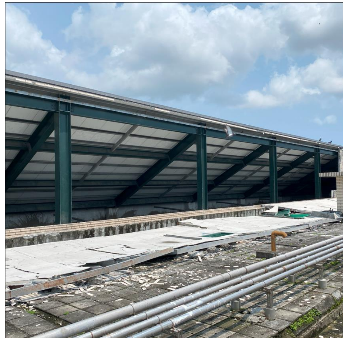
Collapsed windproof walls, composed of LWAC (rooftop)
