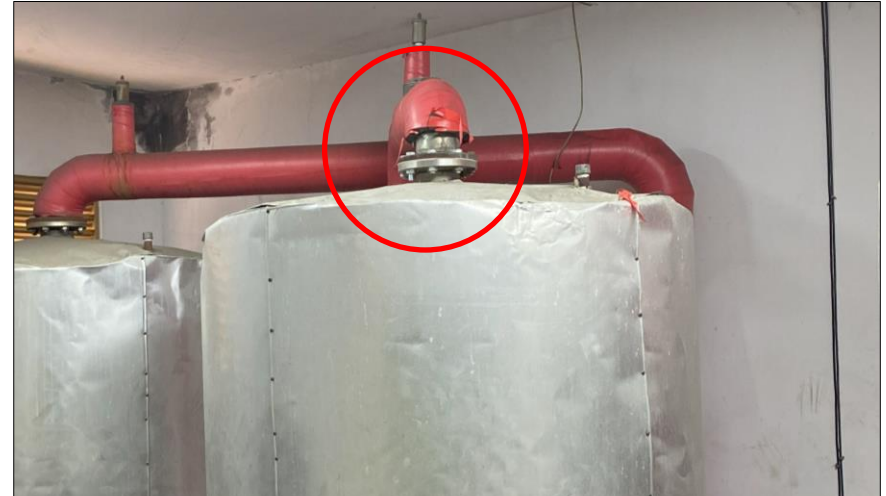
Damaged piping joints connected to the hot water tank in Bldg. A3 (repaired)
