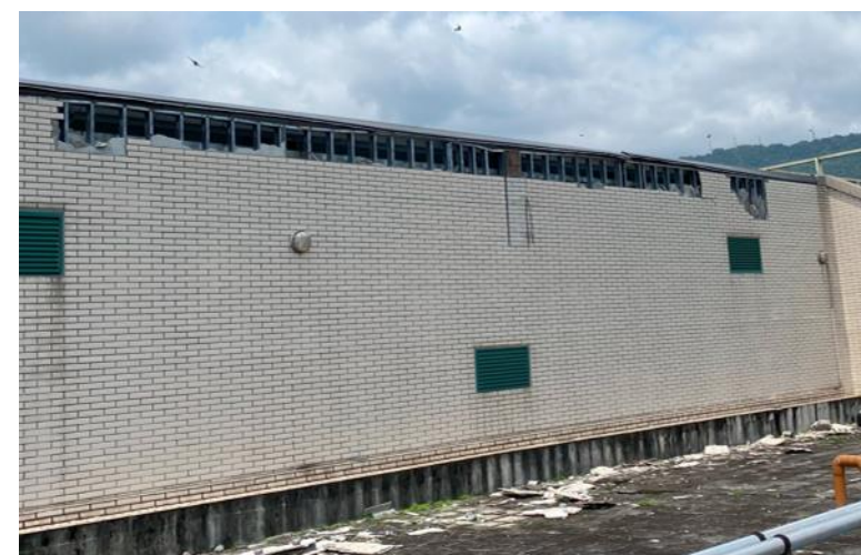
Partially-damaged windproof wall
