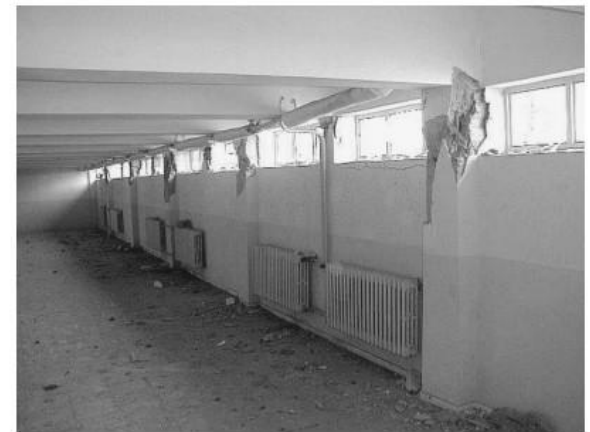
Figure 9. Typical example of captive columns. (Photograph by Mete Sözen)
