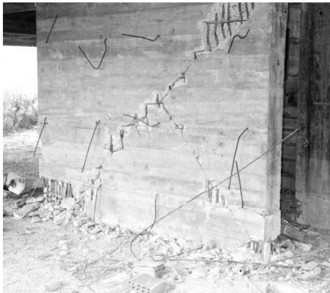
Figure 8. Failure of a shear wall in Bolu.
