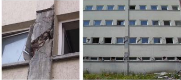
Figure 8. Captive column effect and buckling of longitudinal steel in Bolu (view from the courtyard).
