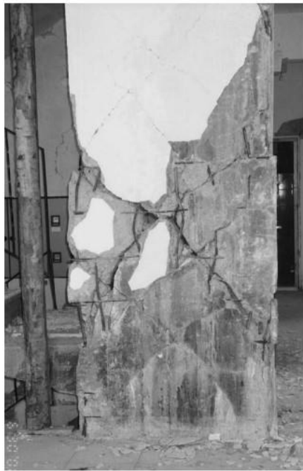
Figure 7. Column failure, Bolu government hospital.
