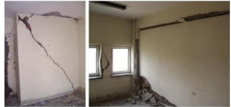
Figure 9. Failure of infill walls.
