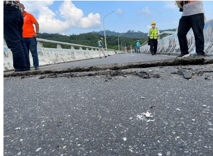
Deck displacement, guardrail and attached pipe broken
