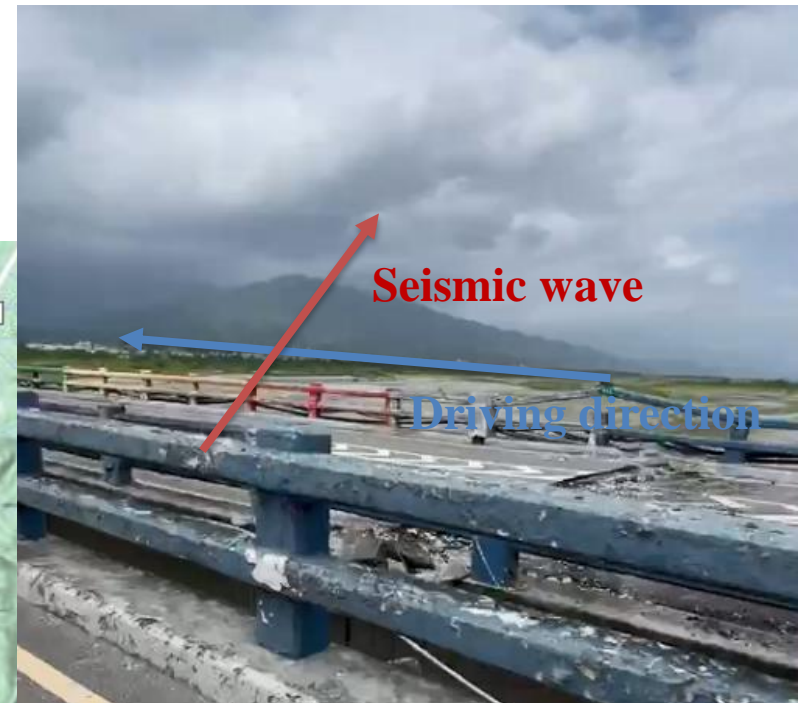
Damage at expansion joint
