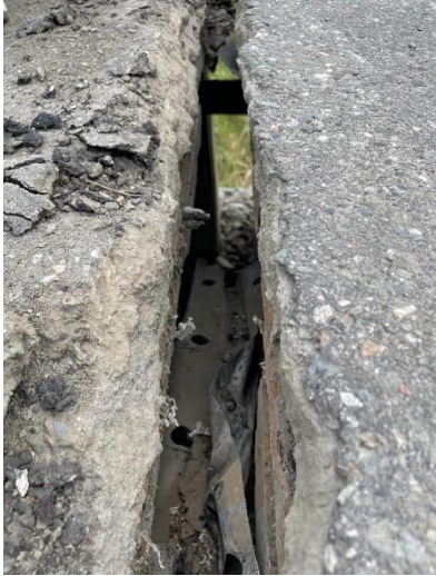
large displacement at expansion joint, support serious damage
