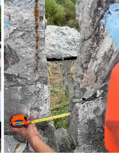
large displacement at expansion joint, support serious damage
