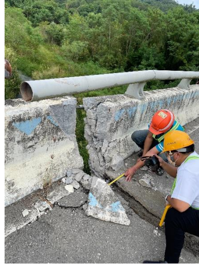
large displacement at expansion joint, support serious damage
