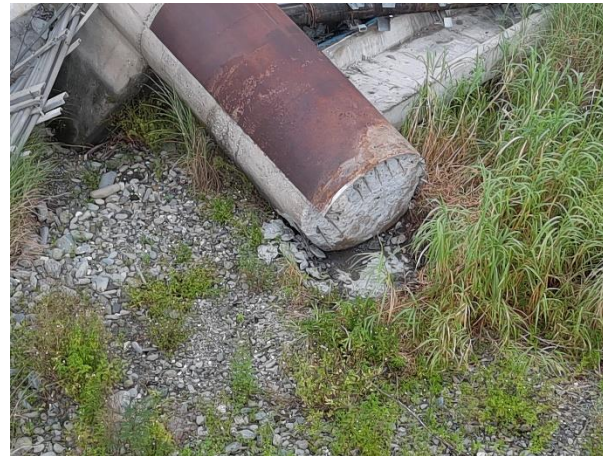
Bridge falling and bridge column fracture
