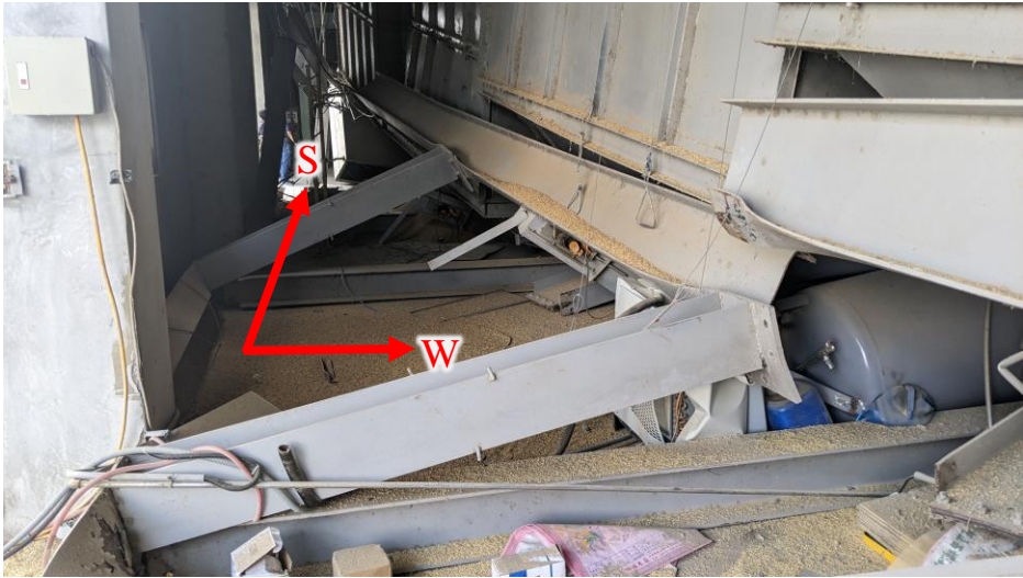
The failure of the supporting frame underneath the tanks led to the grain tanks collapsed toward southwest in 9/17 event.
