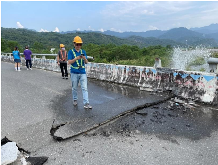
Deck displacement, guardrail and attached pipe broken
