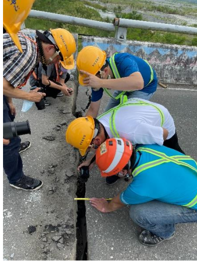
large displacement at expansion joint, support serious damage
