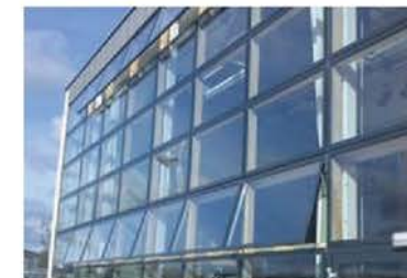
9. MECHANICALLY OPERABLE WINDOW
