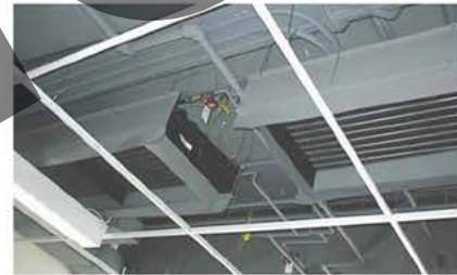
7. ACTIVE CHILLED BEAMS
