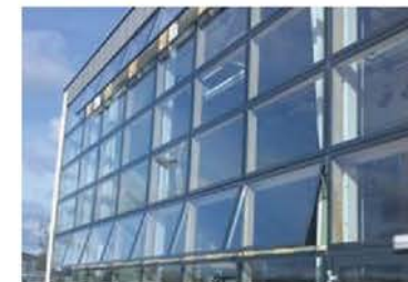
9. MECHANICALLY OPERABLE WINDOW
