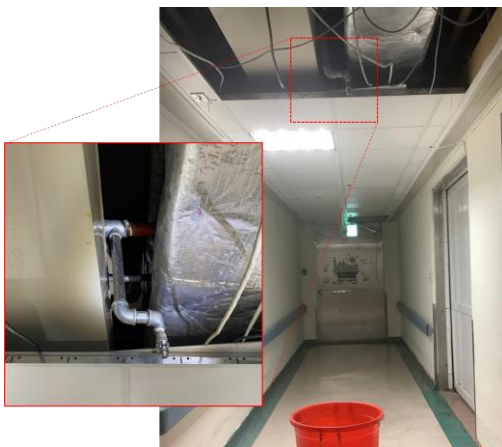
Fig. 41 The damaged piping joint on the fifth floor of Taitung Hospital, Chenggong branch (PGA: 535 gal).
