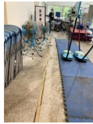
(b) Cracks on north side of the ground.
