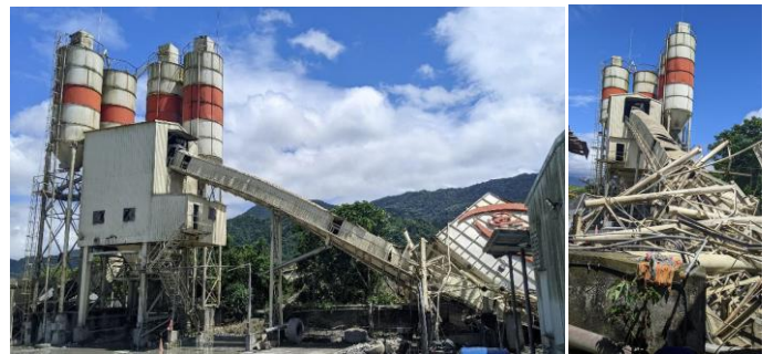
Fig. 32 Da-Yuan quarry storage tank and conveyor belts that collapsed and deformed during the earthquake (PGA: 175 gal).
