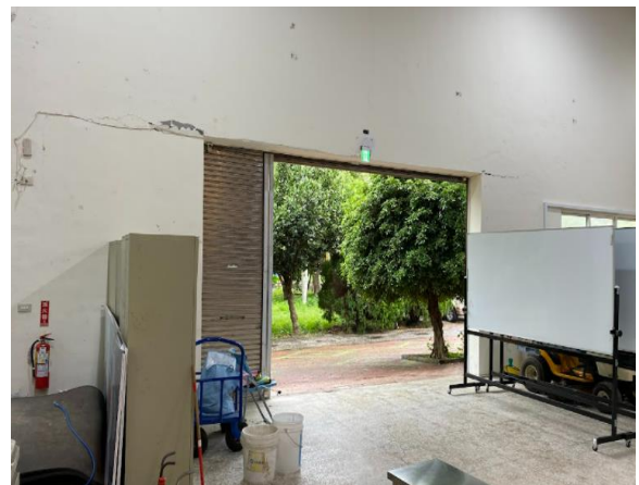
Fig. 23 Horizontal cracks at the top corners of both sides of the door frame at the entrance of Zhongxiao Elementary School (PGA: 401 gal).
