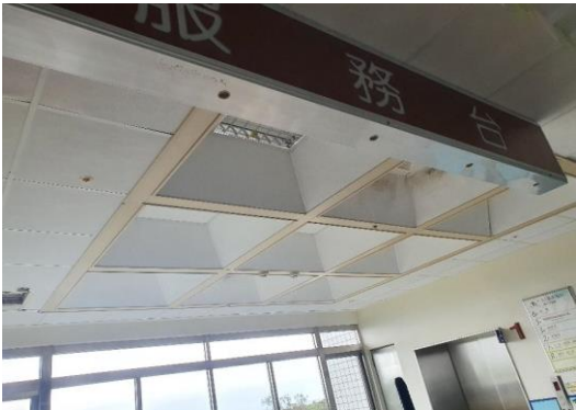
Fig. 34 The specialty ceiling in the first-floor elevator lobby at Taitung Hospital (PGA: 535 gal).
