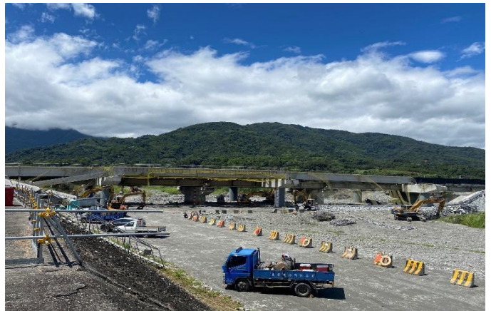
Fig. 28 The east side of the Yuxing Bridge after demolition (PGA: 135 gal).
