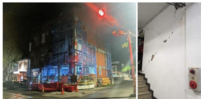
Fig. 48 Dong-He Station, Taitung County Fire Department being retrofitted. The brick wall outside the duty room on first floor was cracked, and the door got jammed (PGA: 409 gal).
