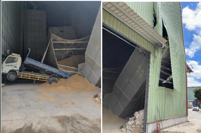
Fig. 30 The Nian-Chang rice mill 15-m-high grain tanks that collapsed westward and collided with the storehouse and trucks (PGA: 140 gal).
