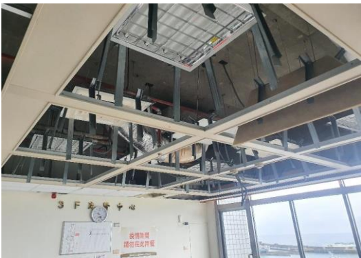
Fig. 35 The damaged specialty ceiling in the elevator lobby on the third floor of Taitung Hospital (PGA: 535 gal).
