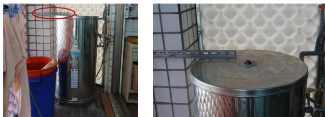
Fig. 46 The damaged heater, which was repaired after the earthquake and strengthened by attaching a steel angle iron at its top, Taitung Hospital. This is not a long-term solution for supporting the weight of the heater (PGA: 535 gal).
