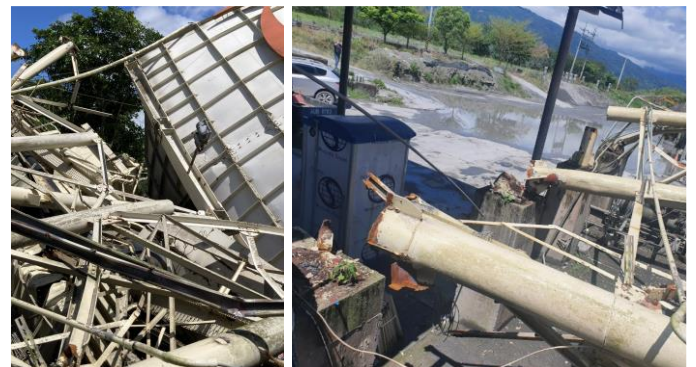
Fig. 33 Top and bottom ends of Da-Yuan steel columns that were ruptured neatly (PGA: 175 gal).
