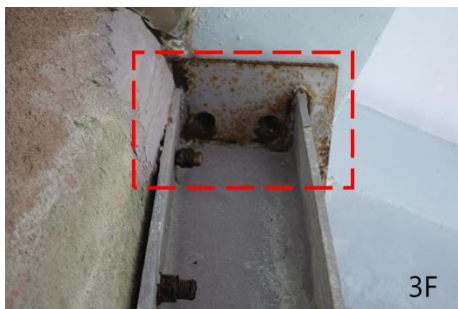
Fig. 20. Top bolts of the added steel column on the 3rd story that had fallen and were missing, CGES building (PGA: 515 gal).
