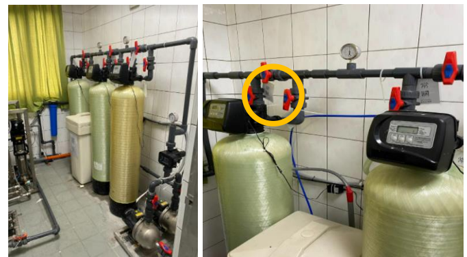
Fig. 44 The marked pipe was sheared off, Taitung Hospital (PGA: 535 gal).
