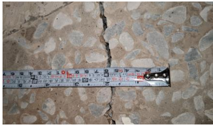
(a) Crack width
