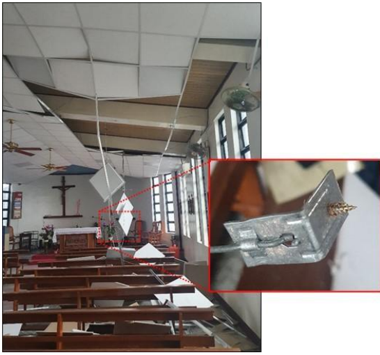
Fig. 40 Damaged to exposed ceiling in Yong-Fu Presbyterian Church (PGA: 336 gal).
