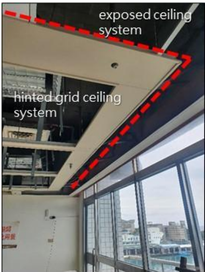
Fig. 35 The damaged specialty ceiling in the elevator lobby on the third floor of Taitung Hospital (PGA: 535 gal).
