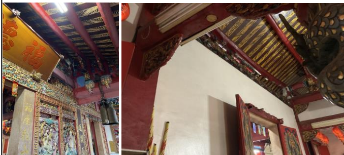
Fig. 26 Small statues instead of walls connect the roof and the beam above the front door of the Fude Temple, resulting in a sudden reduction in strength (PGA: 524 gal).
