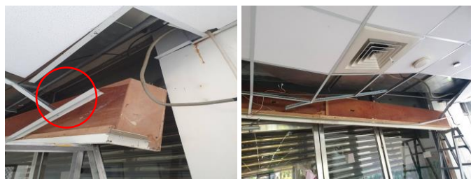
Fig. 50 Failure of an air-conditioning box and suspended ceilings, Yuli Hospital (PGA: 135 gal).
