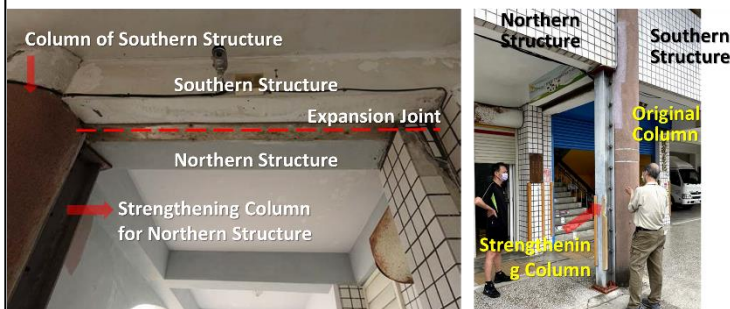
Fig. 19 Expansion joint connecting the northern and southern parts of the western CGES building (PGA: 515 gal).
