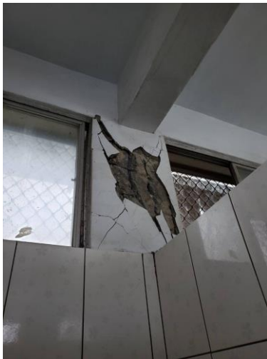
Fig. 18 Damaged short column of the CGES lavatory (source: Taitung County Government).
