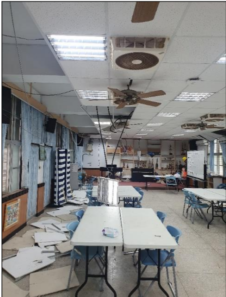
Fig. 37 Damaged exposed ceiling at Zhongxiao Elementary School (PGA: 401 gal).
