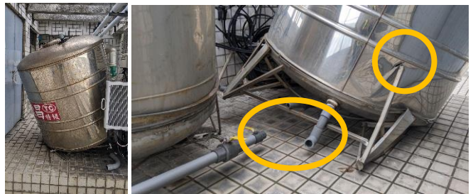
Fig. 43 Tilted water tank due to failure of the stand underneath it, Taitung Hospital (PGA: 535 gal).
