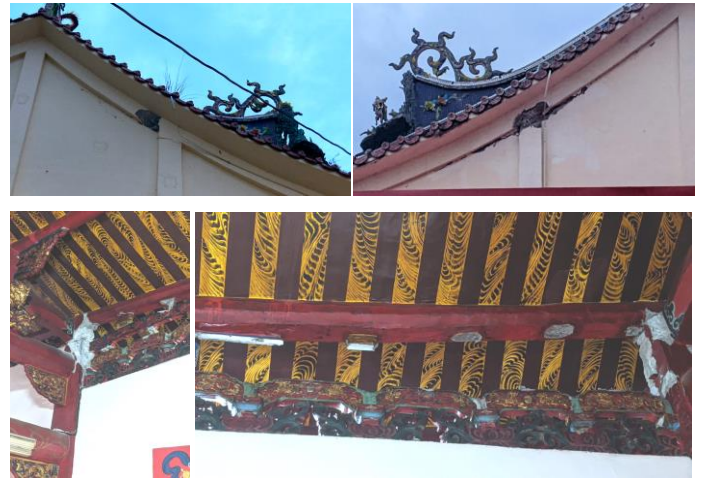
Fig. 27 Damaged beam-column joints underneath the roof and the cracked diaphragms, Fude Temple. The small statues between the beam and the roof fell apart to the ground (PGA: 524 gal).
