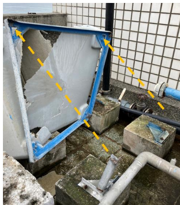
Fig. 45 Seriously damaged FRP expansion water tank on the roof of the Taitung Hospital, Chenggong branch (PGA: 535 gal).
