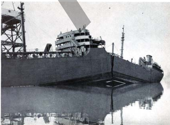
FIGURE 11—View of S. S. Selenia after splitting in two at her outfitting dock.
