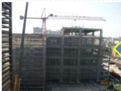
102/03/07 RF澆置、R1F吊裝
