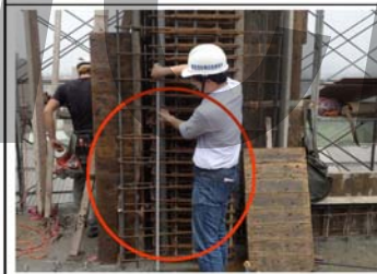
柱牆鋼筋
