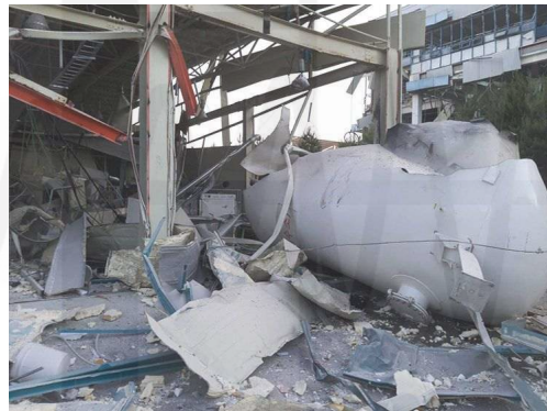
Fig. 5. Hydrogen storage tank accident (Kim & Kim, 2019).
