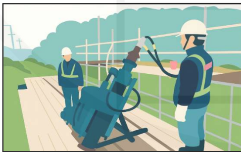
Fig. 5. Scaffolding work platforms and drilling equipment installed on the embankment slope.
