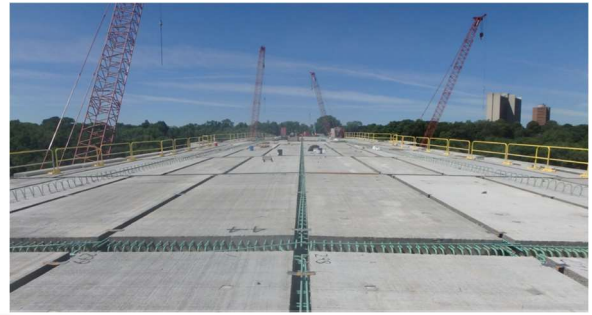
Fig. 3. Closure region between precast bridge deck panels.
