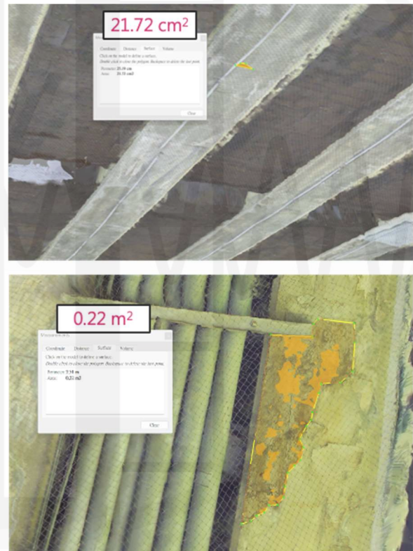
Fig. 4. Smart bridge inspection framework.
