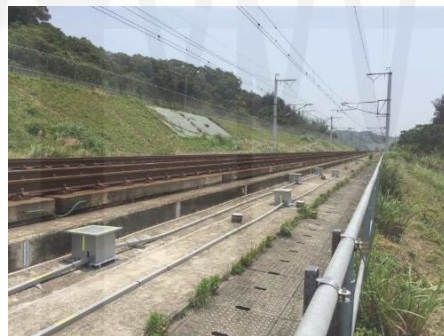
Fig. 1. Real-time monitoring of a track-embankment improvement project in Miaoli, Taiwan.
