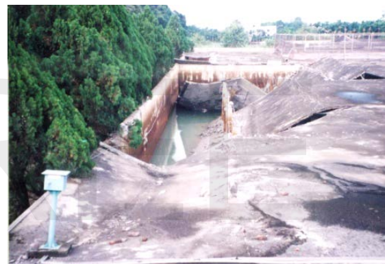
Figure 4. Damage to one of the two clear water tanks of FY1 during the Chi-Chi earthquake
