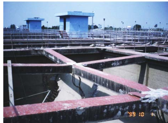
Figure 3. Damage to one of the three sedimentation basins of FY1 during the Chi-Chi earthquake
