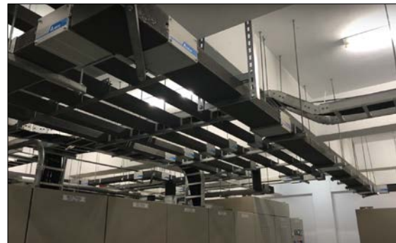
Figure 1. The suspended busway system
