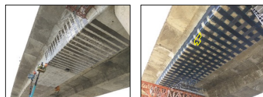
Figure 1. Bridge damage conditions and CFRP reinforcement sheets for shear strengthening.
