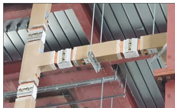
Figure 4. The cast resin busway system
