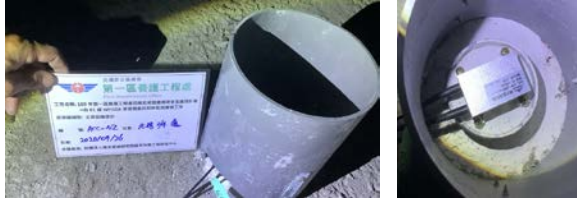
Figure 4. Installation of the optic fiber accelerometer on the main girder
