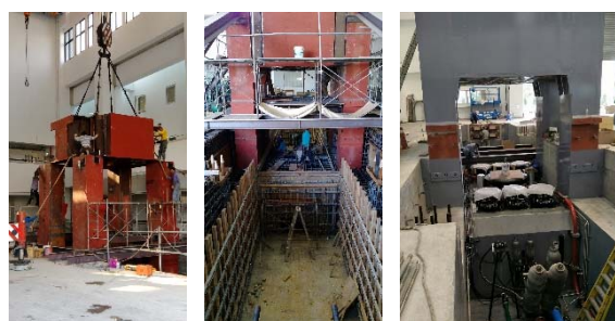
Fig. 11. Progress of construction of the BATS.
