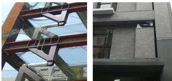
Figure 3 Practical cases of damper configurations in Taiwan.
