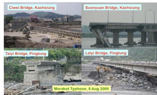
Figure 1. Bridge failure due to scour in Taiwan
